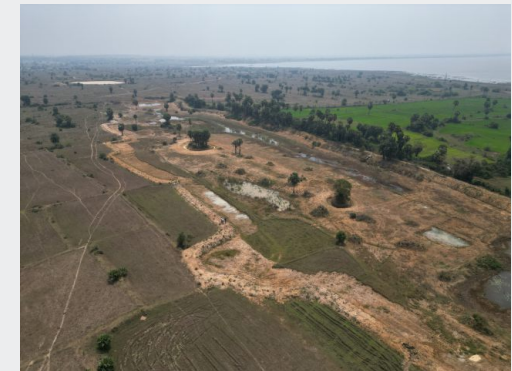
Foreshore & offshore embankments created with bunding work
