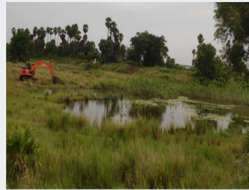
Removal of the weeds and shrubs
